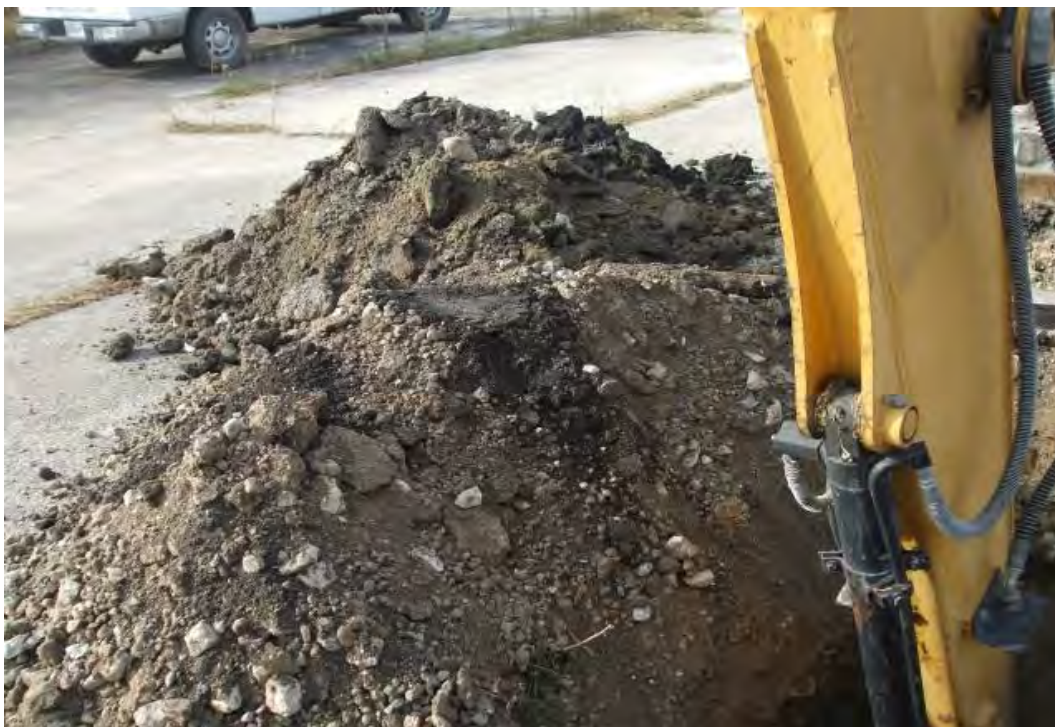
Photograph No. 15 Excavated Granular Soils from TP-10
