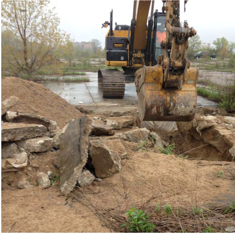
Photograph No. 5 – Excavating LT-4
