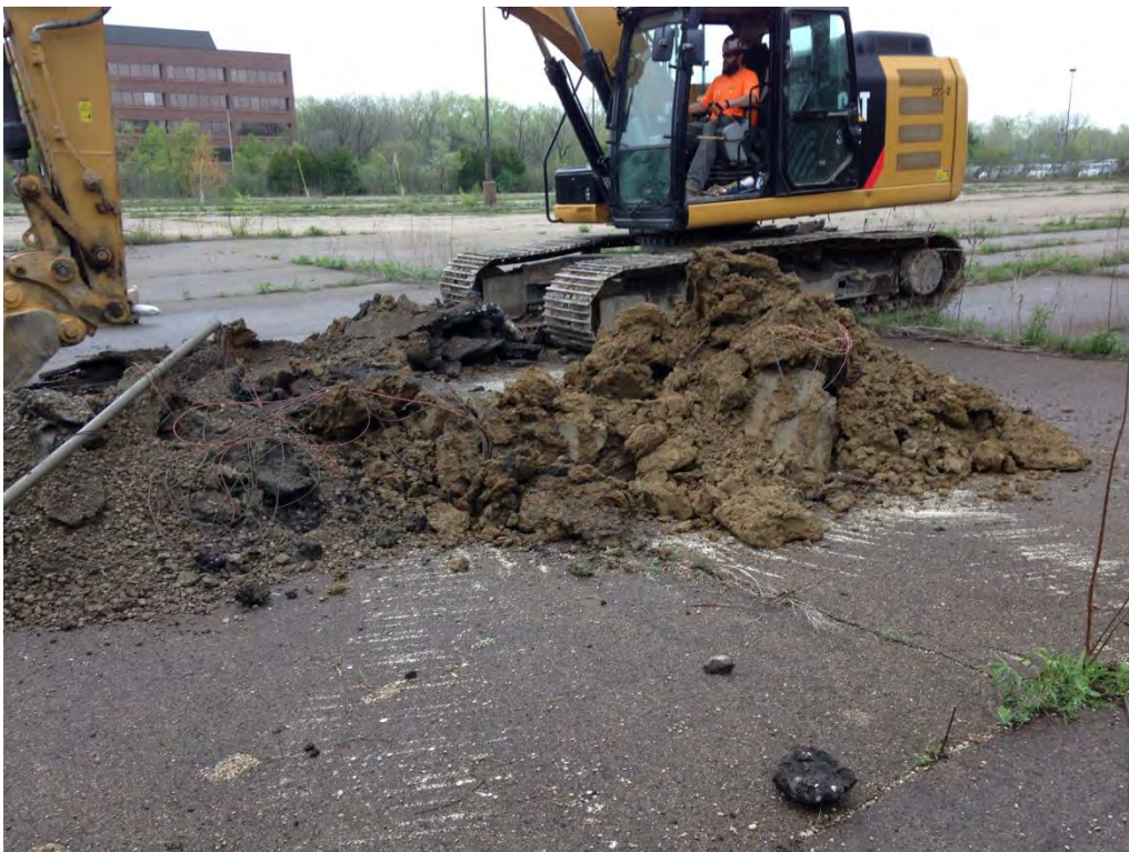
Photograph No. 12 – Excavated Wiring from LT-8
